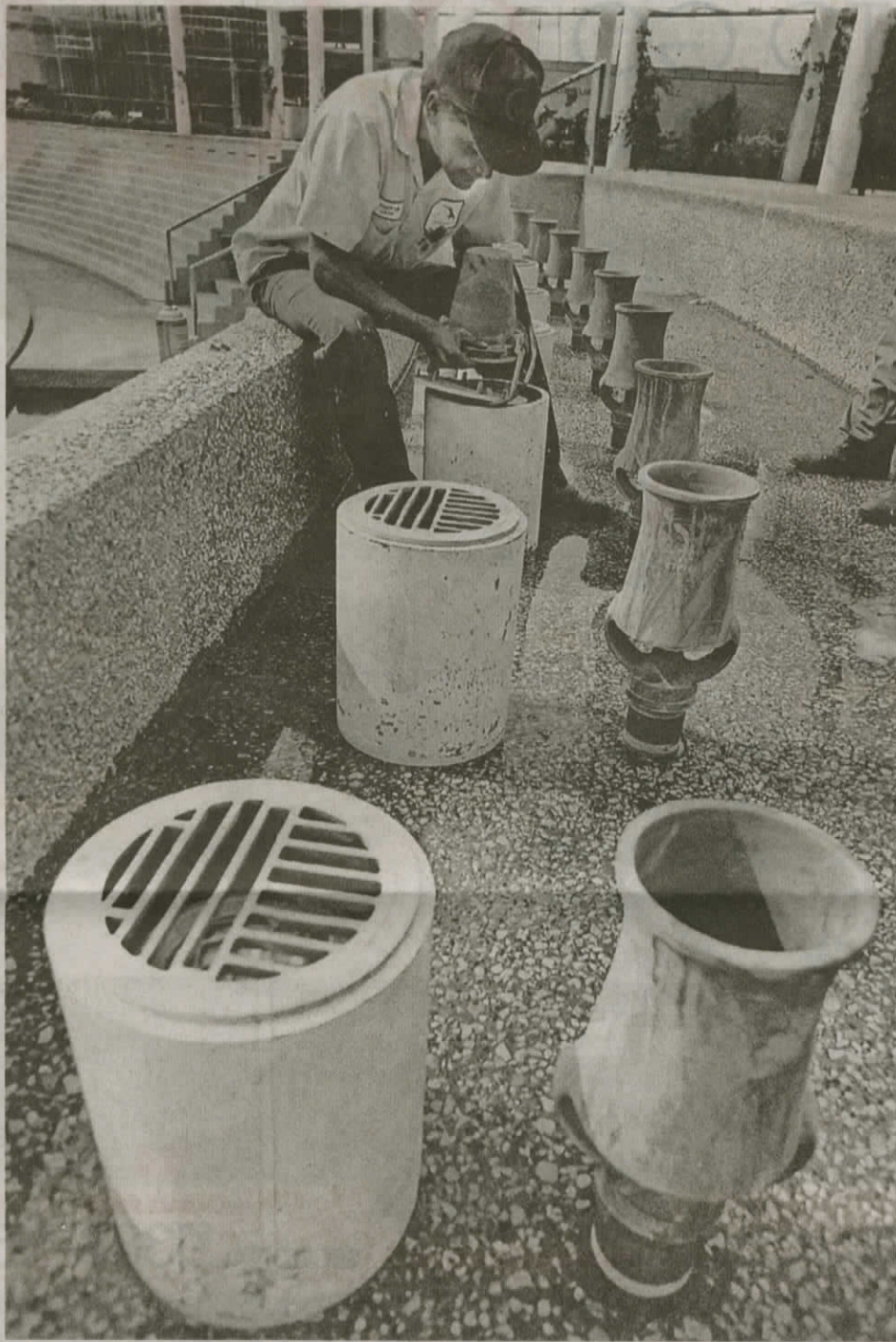
Alex Ronje, employee with the Bayfront Plaza Convention Center maintenance department, replaces one of the burnt-out bulbs in the lights that illuminate the Corpus Christi Watergarden in October 1989. CARLOS MORENO/CALLER-TIMES FILE
