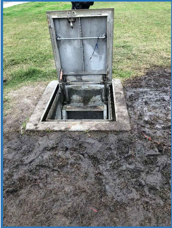
Ground Level Personnel Hatch
