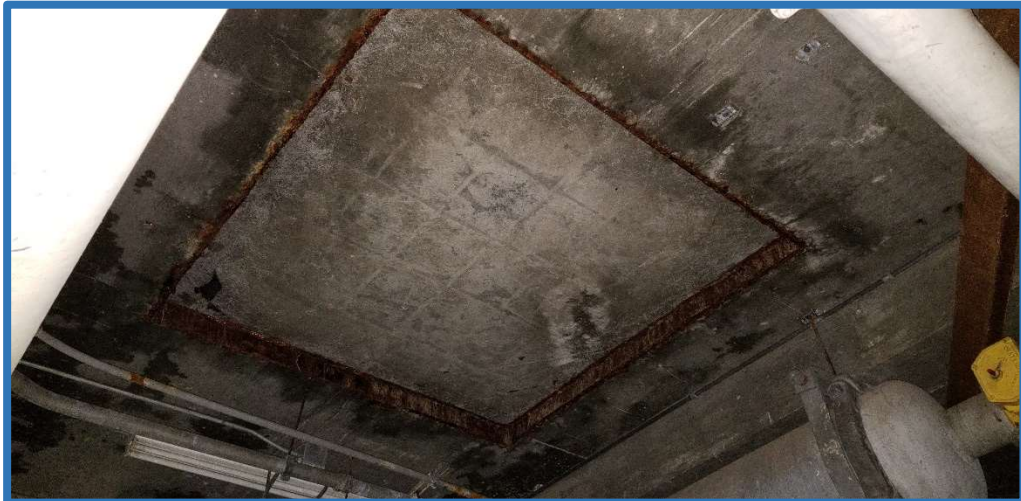
Concrete Equipment Hatch in Vault Roof
