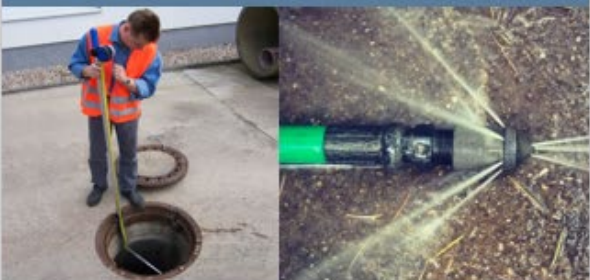
H. SEDIMENT MONITORING + CLEANING
