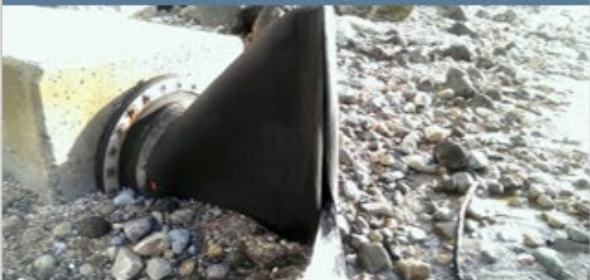
C. TIDE GATES/VALVES (BACKFLOW)
