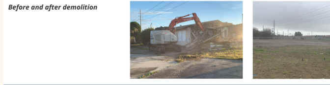
Before and after demolition
