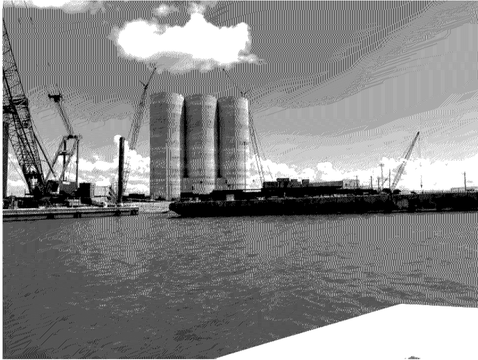
Photo 3- Photo showing northwest of proposed discharge location.
